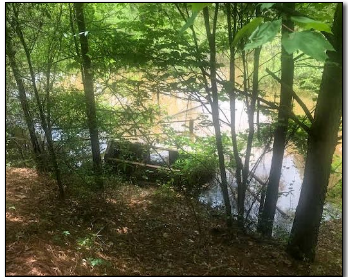
Repaired blown out dam at the mill pond
